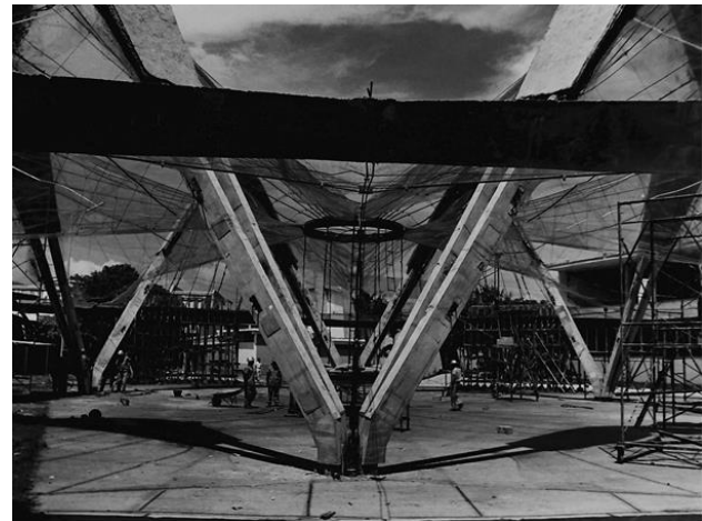
Fig. 6 Supporting on steel arches (Ref.1)
