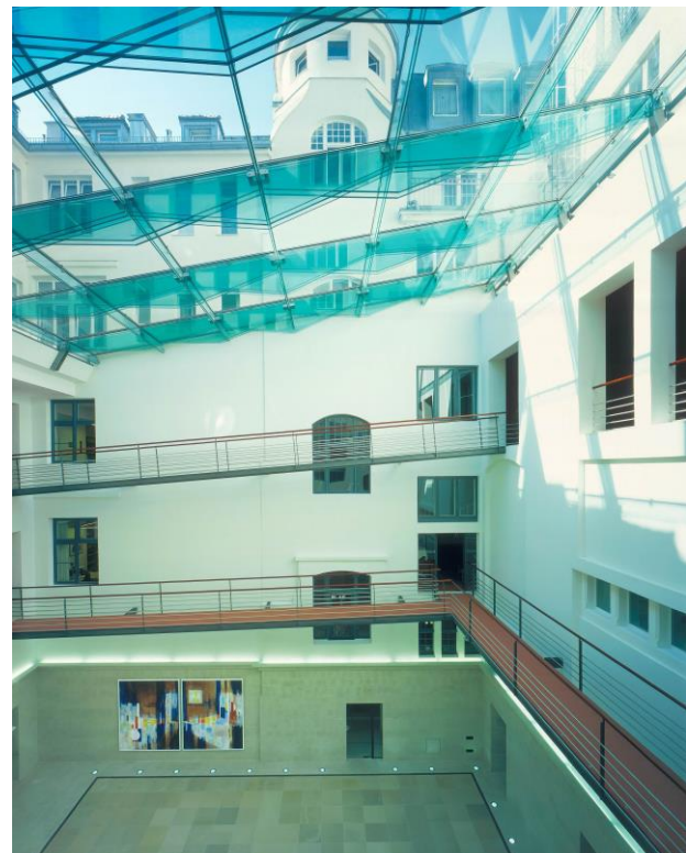
Fig. 1 Segmental Glass Beams in Load-Bearing Roof Structure, Chamber of Industry and Commerce (IHK) Munich, Germany.
