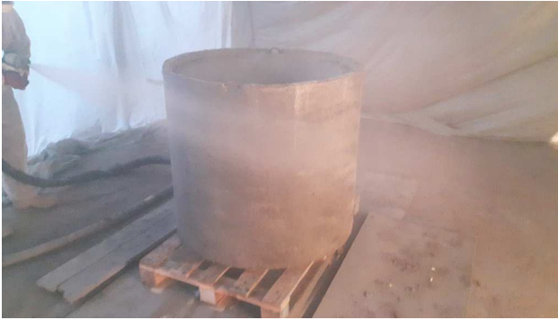
Fig. 5 Spraying polyurea coating system on concrete ring
