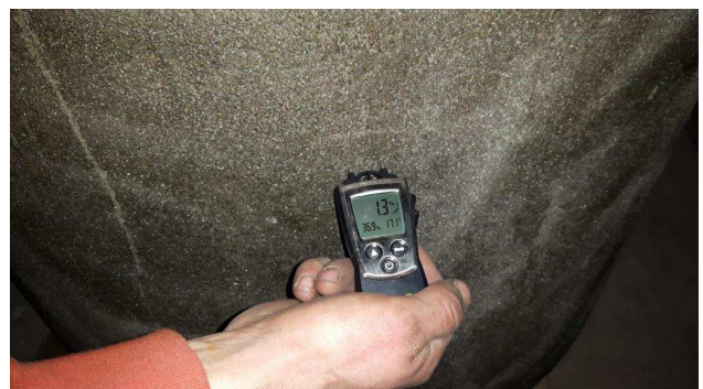
Fig. 4 Measurement of temperature and humidity before application polyurea coating
