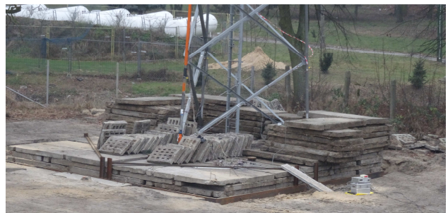
Fig. 10 Final foundation with asymmetric mass distribution
