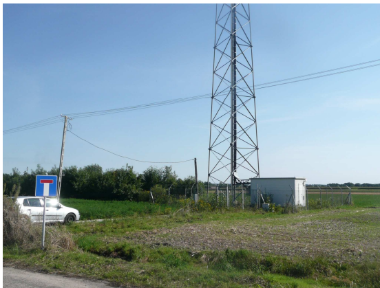
Fig. 2 Unfavorable location of the tower structure: close neighborhood of the medium voltage transmission lines
