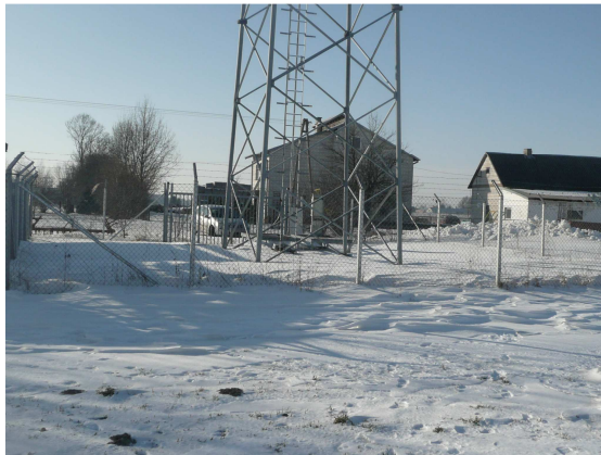
Fig. 1 Unfavorable location of the tower structure: close neighborhood of the buildings
