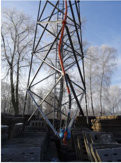
Fig.16 Buckling of the tower leg in section S-7 (second tower)
